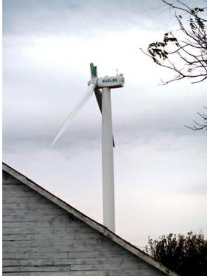
Figure 17. Blade failure at the stem on a 140 feet radius wind turbine at Wyanet, Bureau County, Illinois, October 22, 2008. The blade landed 150 feet from the base of the structural tower.
