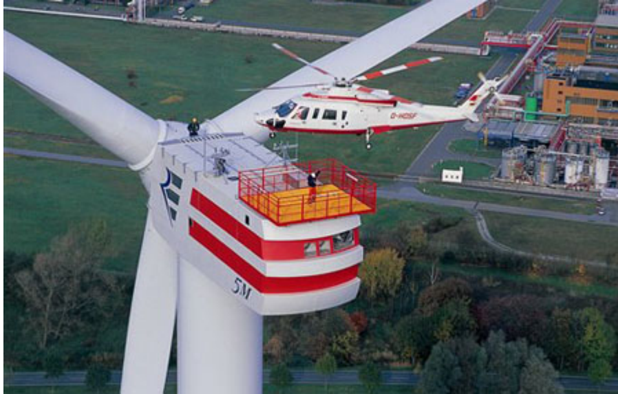
Figure 2. Maintenance access of a wind turbine's nacelle through the use of a helicopter.
