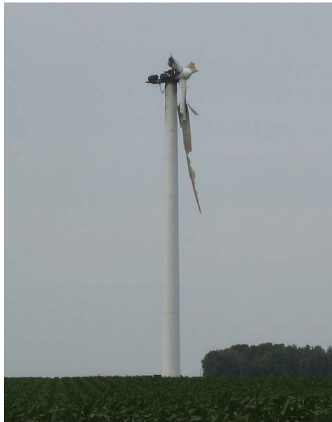
Figure 7. Lightning strike damage on a wind turbine in southern Minnesota, USA, resulted in the destruction of the nacelle and the rotor blades.
