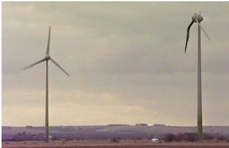
Figure 28. Blade failure due to possible ice shedding from one blade unto another or a manufacturing defect, Conisholme, Lincolnshire, UK.
