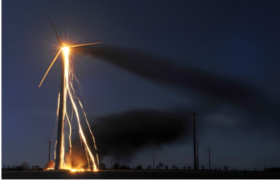
Figure 5. Wind turbine with ignited leaking lubrication oil near Uelzen, Lower Saxony, Germany, December 2, 2009. Source: DPA.
