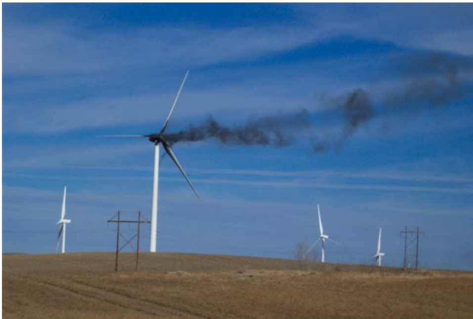
Figure 6. Wind turbine nacelle fire near Bloomingdale, Minnesota, USA, 2008.
