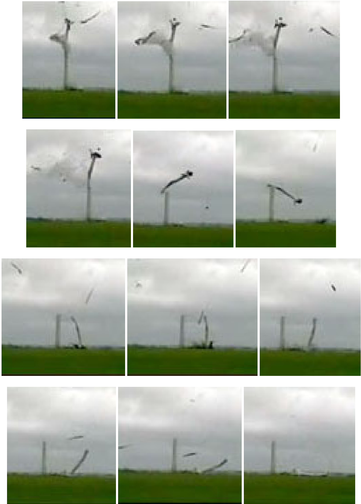
Figure 12. Runaway turbine disintegration clip sequence from video caused by failure of
