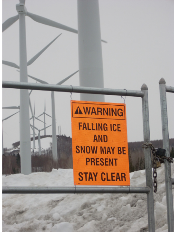
Figure 30. Judicious warning about ice shedding and limited access at a wind turbine site, USA.
