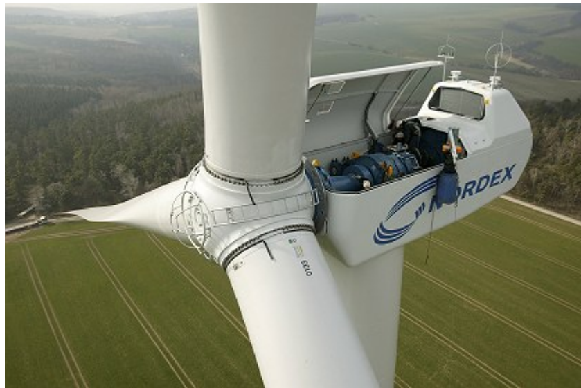
Figure 1. Maintenance at wind turbines nacelles involves work at about 100 meters height. Source: Getty, Nordex.
