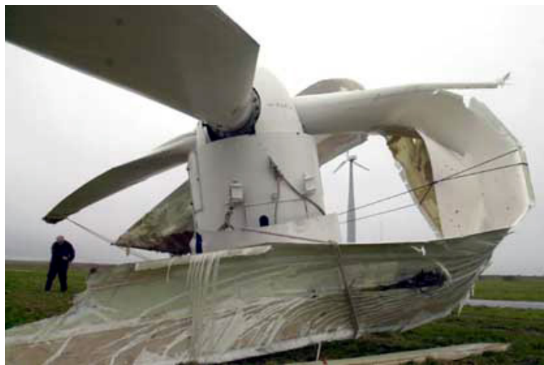
Figure 19. Structural collapse of a wind turbine in a 2002 storm. Source: Der Spiegel, DPA.
