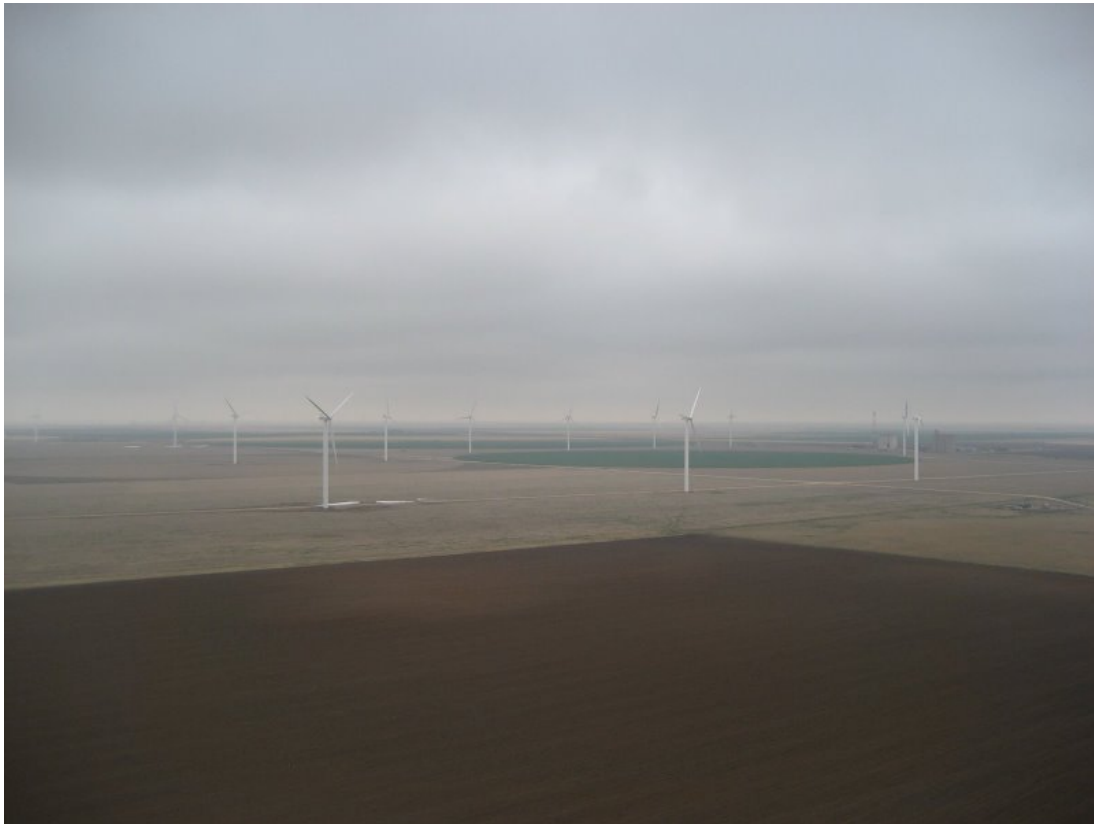
Figure 23. Recall and replacement of rotor blades in a wind farm due to a manufacturing defect, USA.
